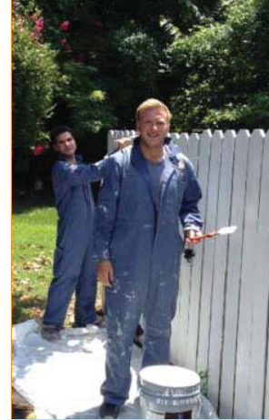
AmeriCorps volunteers make repairs and paint at WCCS.
